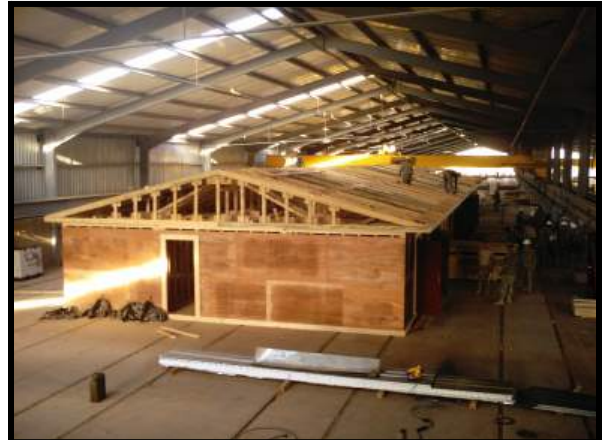
The front side of building number one
