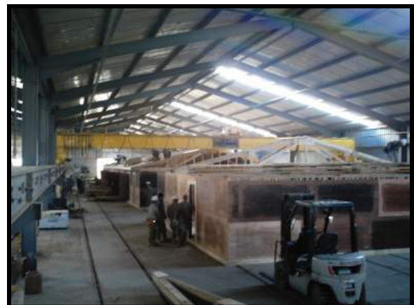
The back side of building number two
